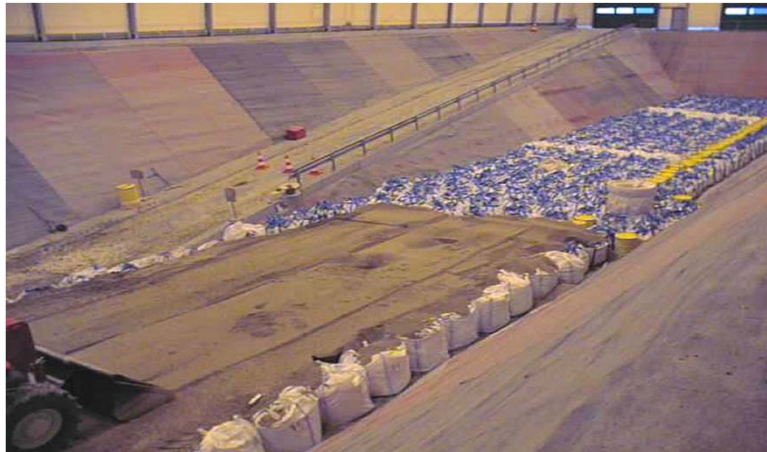
Very low level waste repository, Morvilliers, France
