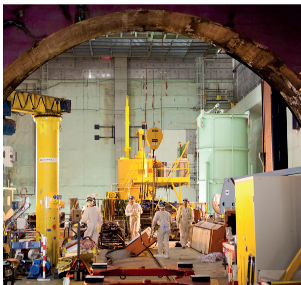
Deconstruction site at the Chooz A power plant: deconstruction of the cavern
