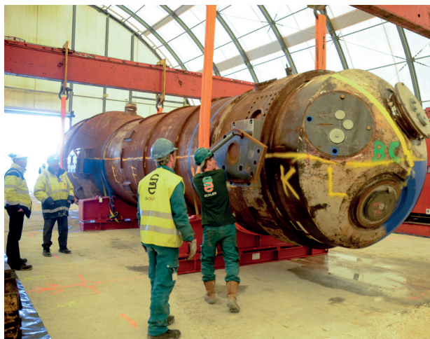
Disposal of a steam generator from the Chooz A power plant in Cires.
