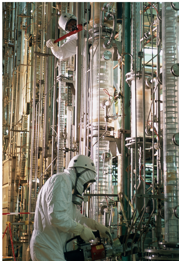
Dismantling of a prototype facility for pulsed column solvent extraction (INB57) at the CEA Fontenay-aux-Roses facility
