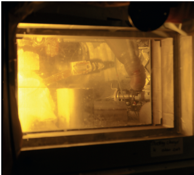
Cleanup of a shielded cell from the Cyrano line at the CEA Fontenay-aux-Roses facility
