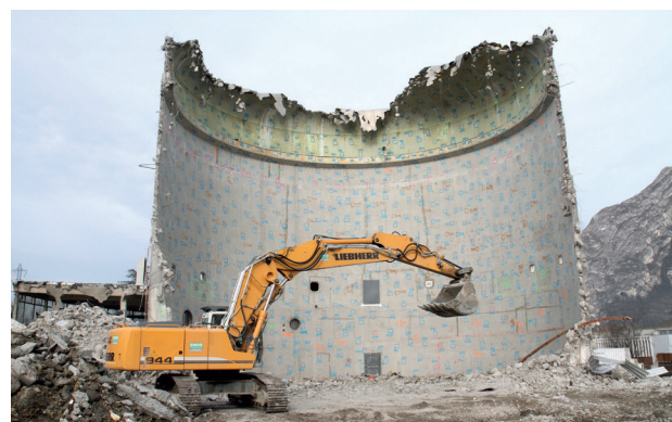
Dismantling of the Siloé reactor at the CEA Grenoble facility
