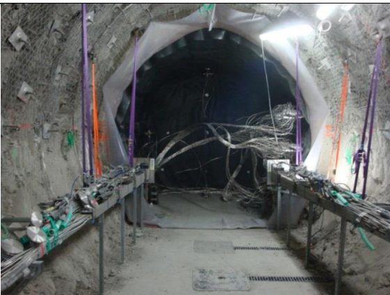
Seal core instrumentation before concrete casting in the injection chamber
