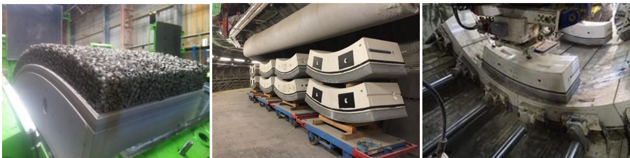
Figure 3 Prefabrication and installation of VMC liner segments in one of the 3 sections of GVA2
