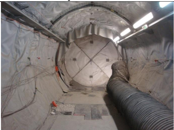
Installation of membranes at the core/retaining plug interface (before concrete casting)
