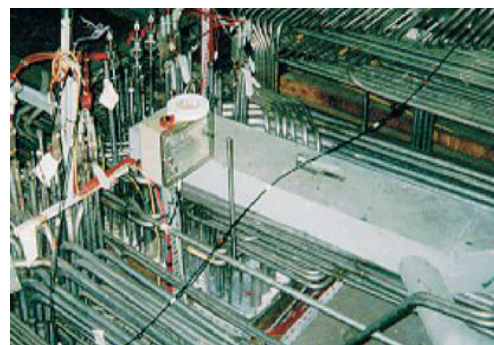
► Figure 1: Inspection of a contaminated pipe system using an OSL system
