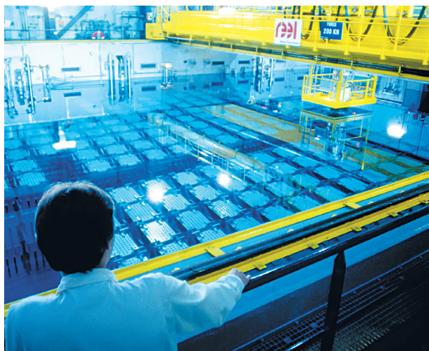
Spent fuel storage pool at the Orano reprocessing plant in La Hague
