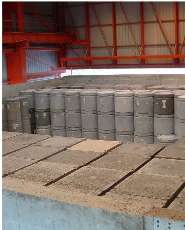
Disposal of waste packages in the disposal vaults at the Aube disposal facility (CSA)
