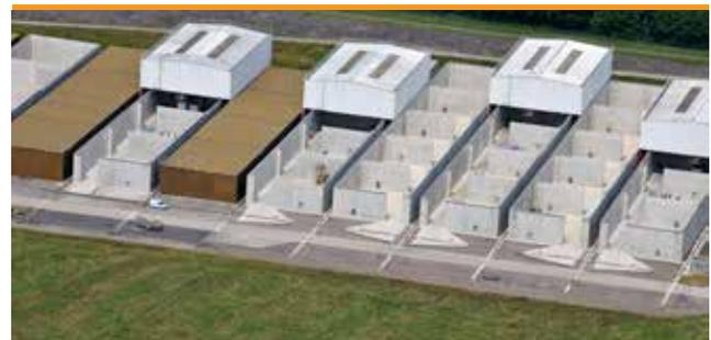
With a surface area of 95 hectares and an authorized disposal capacity of 1,000,000 m<sup>3</sup>, this facility, dedicated to the disposal of short-lived low-and intermediate-level waste, has been in use since 1992. It took over from the Manche Disposal Facility, building on the 25 years of experience already accumulated.
