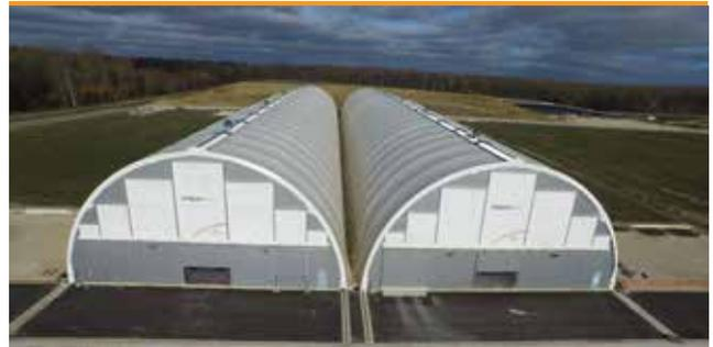
With a surface area of 45 hectares and an authorized disposal capacity of 650,000 m<sup>3</sup>, this facility has been used for the receiving and disposal of very low-level waste since 2003. It has also been used for the collection and storage of waste from non-nuclear power activities since autumn 2012 and for waste sorting and treatment since 2016.
