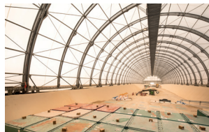
Industrial Facility for Nuclear Waste Collection, Storage and Disposal (Cires)
