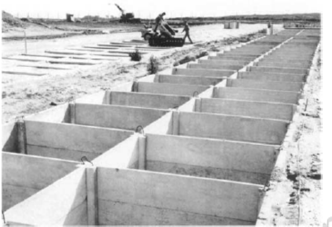
Concrete trenches under construction (1969)
