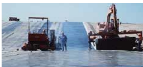
Laying a strip of geomembrane. Strips are welded together.
