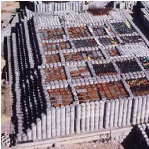
Photo of a disposal structure during the operating phase (circa 1990)
