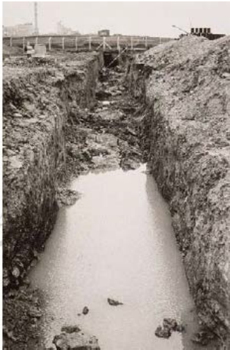
Ordinary disposal trench (1969)
