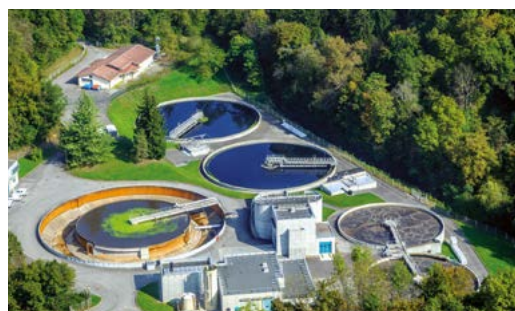
Examples of site development work
