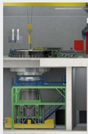
Reception and offloading of transport containers for ILW-LL waste packages
